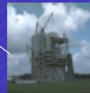
Component Test Facility/Test Stands (SSC)
